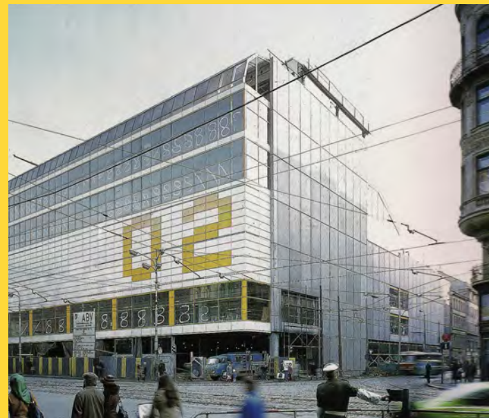
Fig. 3) Máj department store after completion. Prague, Czech Republic. (private archive of Miroslav Masák)
