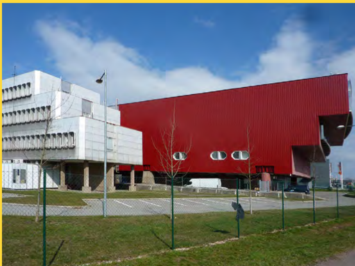
Fig. 5) Telephone exchange stations in Hradec Králové. Czech Republic. (photo Lenka Popelová 2019)
