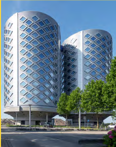
Fig. 1) Sugarcity. The two sugar silos after the conversion into an office complex. Haarlemmermeer, Netherlands. ( commons.wikimedia. org/wiki/File:Halfweg,_ SugarCity_ industri%C3%A8le_ evenementenlocatie_ IMG_0282_2019- 06-30_09.49.jpg ), 4.0 International Public Licence Michielverbeek 2019)
