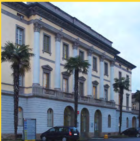
Fig. 1) Building of the former padiglione dei Tranquilli, now headquarter of the socio-educational centre, the Local Health Company rehabilitation centre and the dialysis assistance centre of the Ospedali riuniti, seen from inside the courtyard. Bergamo, Italy. (Archivio fotografico ASST Papa Giovanni XXIII, 2021)
