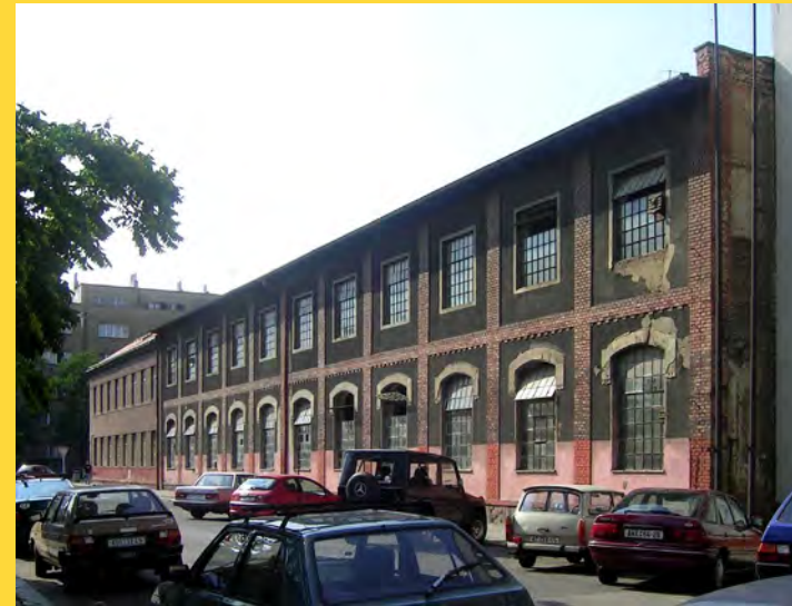
Fig. 16) Former machine works Rossemann & Kühnemann, now DOX Centre for Contemporary Art in Holešovice, Prague, Czech Republic. (photo Vladislava Valchářová 2004)
