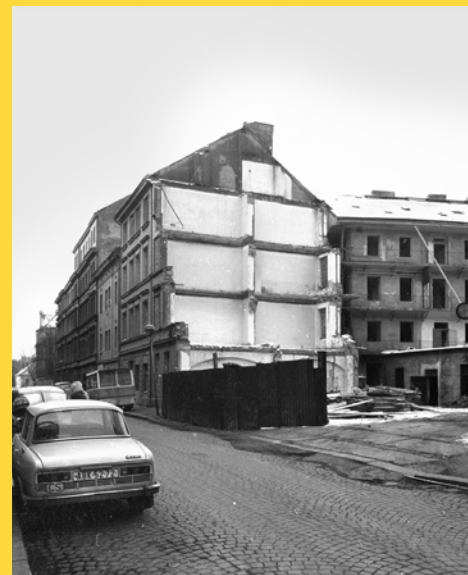
Fig. 3) Demolition of neglected tenement buildings prior to the construction of the Public Transit Company's dispatching centre in Prague, Czech Republic. (archive of the Prague Public Transit Company)
