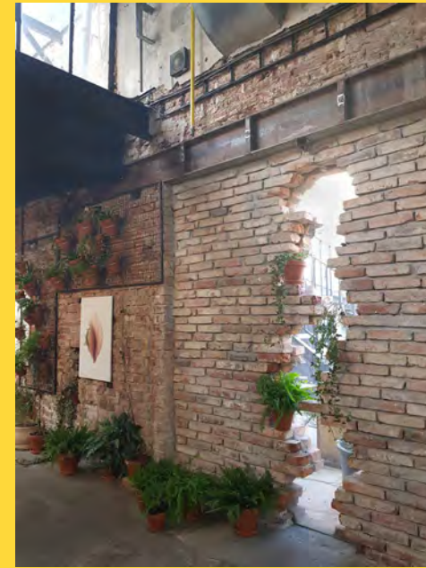
Fig. 3) Interior of Vnitroblok, an industry in Holešovice district converted into an art and entertainment centre by a bottom-up process. Prague, Czech Republic. (photo Naveed Iqbal 2019)
