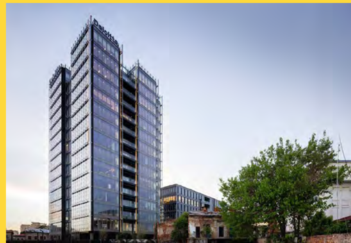
Fig. 7) Contemporary interventions in historic areas: a new office building at Calea Griviței, among the ruins of a large area demolished between 2011–2013. Bucharest, Romania. (photo Alberto Grosescu)
