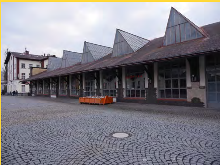
Fig. 1) Exterior of The Prague Market, former Abattoirs, in Holešovice, Prague, Czech Republic. (photo Petr Vorlík 2021)
