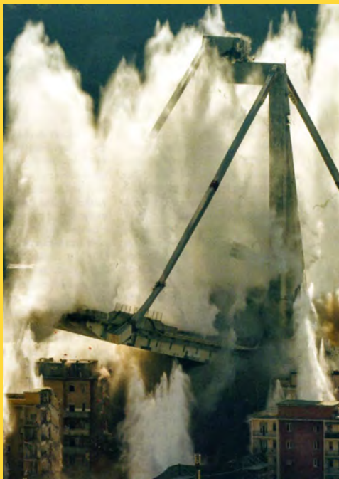
Fig. 1) Demolition of Morandi bridge in 28 June 2019. Genova, Italy. (photo Astrid Fornetti 2019)
