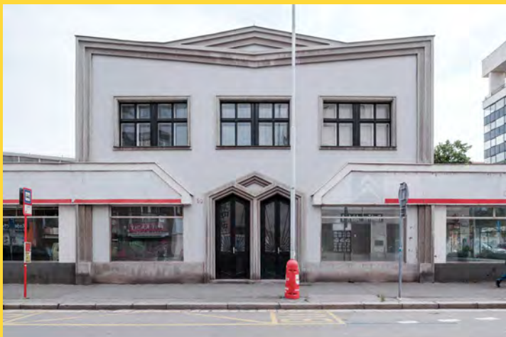
Fig. 1) Materna's Paint Factory before demolitions started. Holešovice, Prague, Czech Republic. (photo Viktor Mácha 2013)
