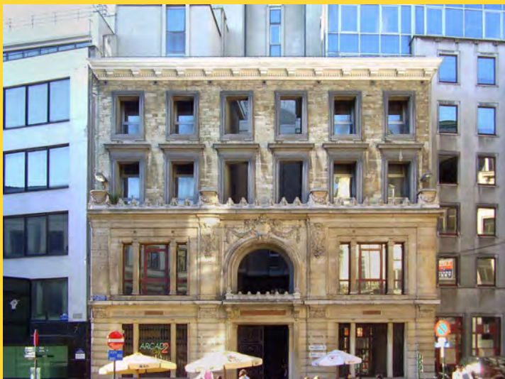
Fig. 1) Façadism in Brussels, Belgium. (< commons.wikimedia.org/wiki/File:Fa%C3%A7adisme_01.JPG >, CC BY-SA 3.0 licence, photo Ben2 2006)
