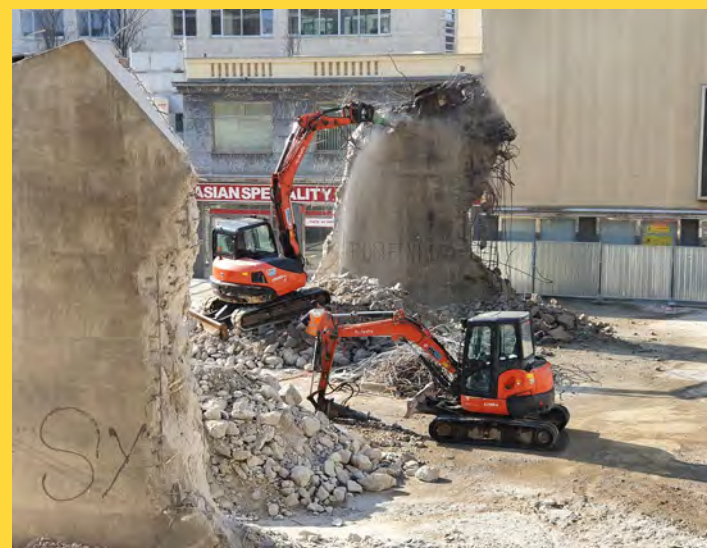
Fig. 8) Demolition of Transgas, Prague, Czech Republic. (photo Petr Vorlík, 2020)
