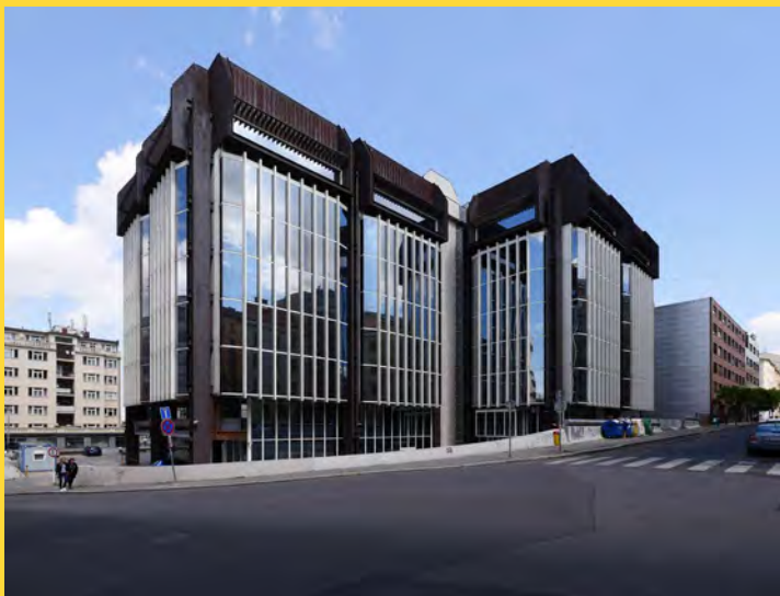
Fig. 5) Transgas before demolition, Prague, Czech Republic. (photo Petr Vorlík, 2017)
