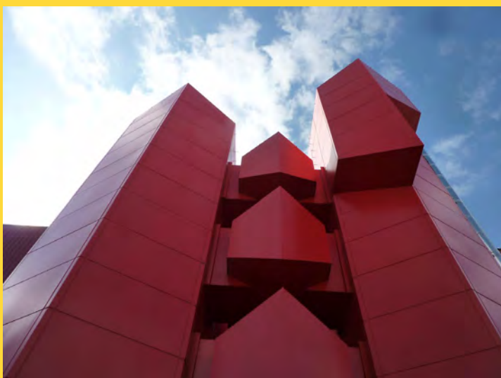
Fig. 6) Telephone exchange stations in Hradec Králové. Czech Republic. (photo Lenka Popelová 2019)
