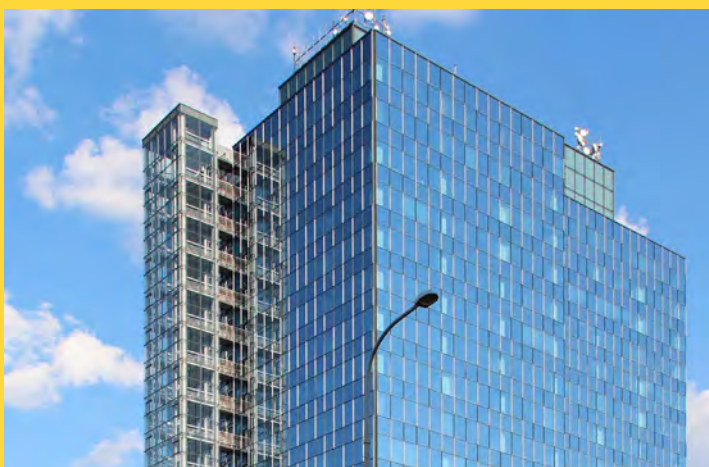
Fig. 10) Kovo building was subjected to a massive interior transformation to achieve higher standards of comfort. Original fire staircase was replaced with new one. Holešovice, Prague, Czech Republic. (photo Petr Vorlík 2018)
