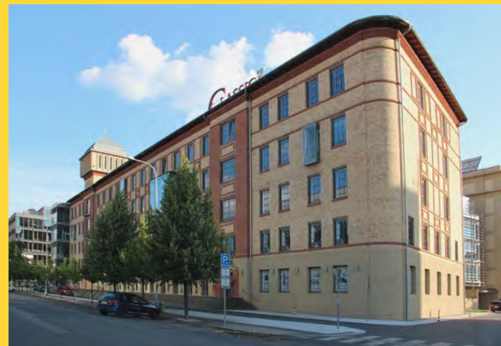
Fig. 7) The Joint-Stock Steam Mill turned into an office building through extensive renovation. Only the tower shows some peculiar features preserved like the timber frame, while finishes has been completely replaced. Holešovice, Prague, Czech Republic. (photo Petr Vorlík 2014)
