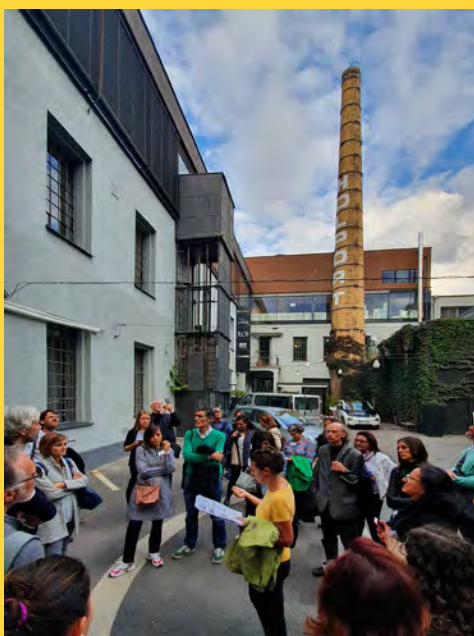
Fig. 6) Former Carl Jerabek Metallwaren Fabrik turned into Design Shop. The chimney have been preserved as a landmark. Holešovice, Prague, Czech Republic. (photo Petr Vorlík 2019)
