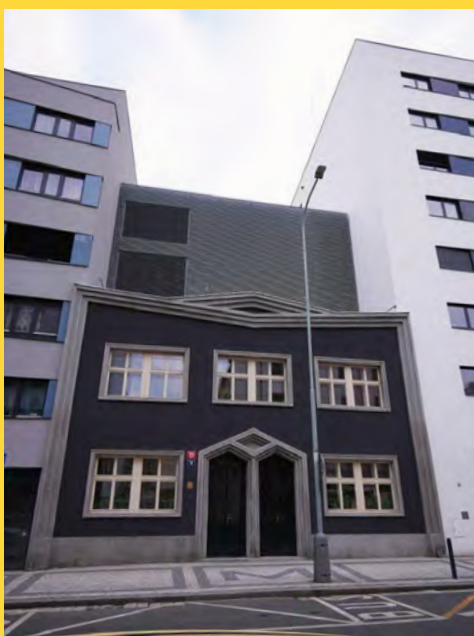
Fig. 2) Materna's Paint Factory. The completely renovated façade has been encapsulated into the new building according to facadism approach. Holešovice, Prague, Czech Republic. (photo Petr Vorlík 2021)
