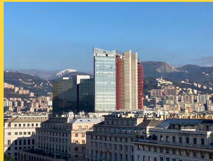
Fig. 7) Corte Lambruschini, the new business centre built after the demolition of a 19 th century building stock – view from the south side. Genova, Italy. (photo Giovanna Franco 2021)
