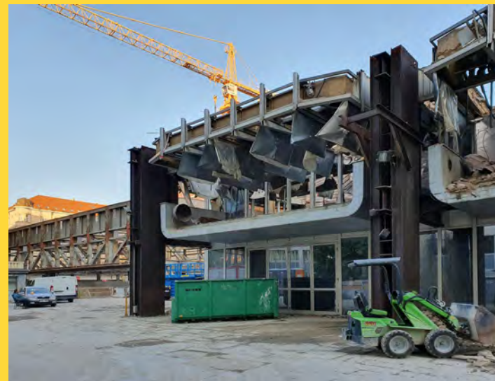
Fig. 7) Demolition of Transgas, Prague, Czech Republic. (photo Petr Vorlík, 2019)
