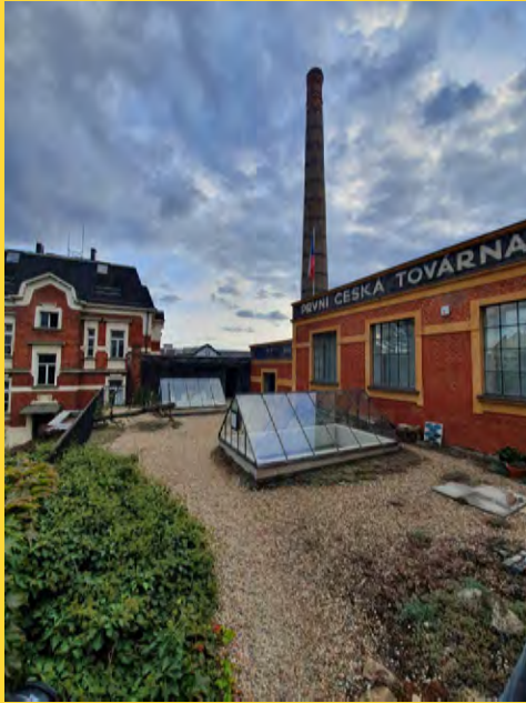
Fig. 5) Factory of water meters in Holešovice converted into Architecture AP Atelier and gallery. Prague, Czech Republic. (photo Petr Vorlík 2019)
