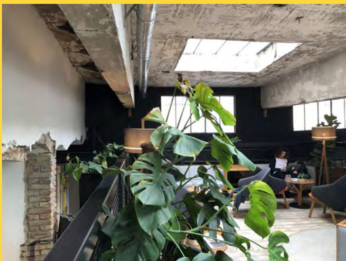
Fig. 2) Vnitroblok complex. The new upper gallery. Prague, Czech Republic. (photo Donatella Fiorani 2019)
