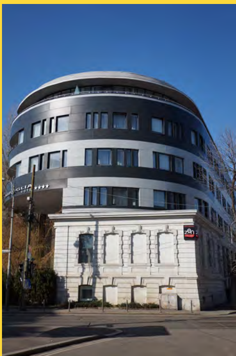
Fig. 6) Contemporary interventions in historic areas: an example of façadism at 59, Vasile Lascar St. Bucharest, Romania. (photo Raluca-Maria Trifa)
