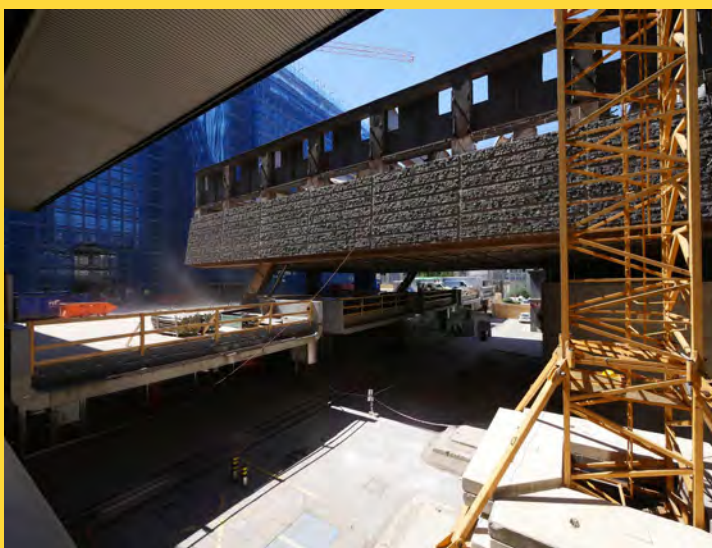
Fig. 6) Demolition of Transgas, Prague, Czech Republic. (photo Petr Vorlík, 2019)
