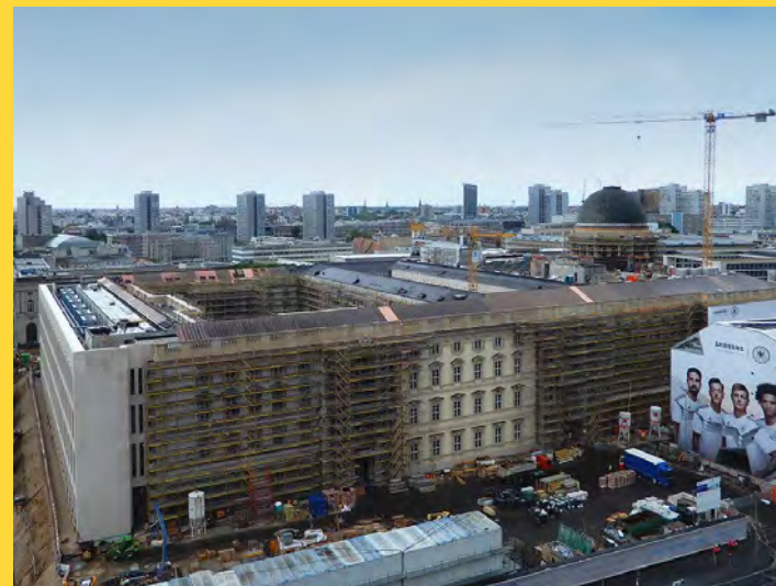
Fig. 7) The Schloss under construction in Berlin, Germany. (photo Stefano Francesco Musso 2018)
